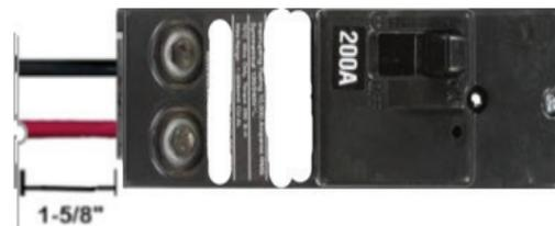
For Siemens Type QN 150A to 200A plug-in main circuit breakers, a minimum of 1-5/8" of unbent feeder wires/leads must be present at the main breaker connection in order for the B3 Bypass to be installed.
